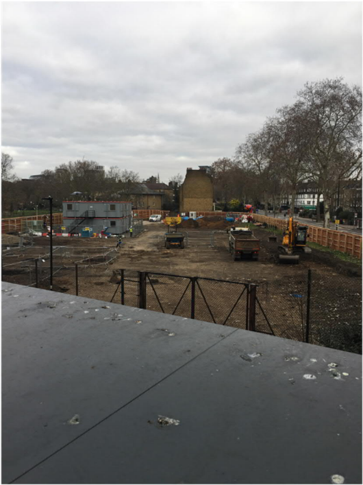
Construction site on Lollard Street opposite the nursery
