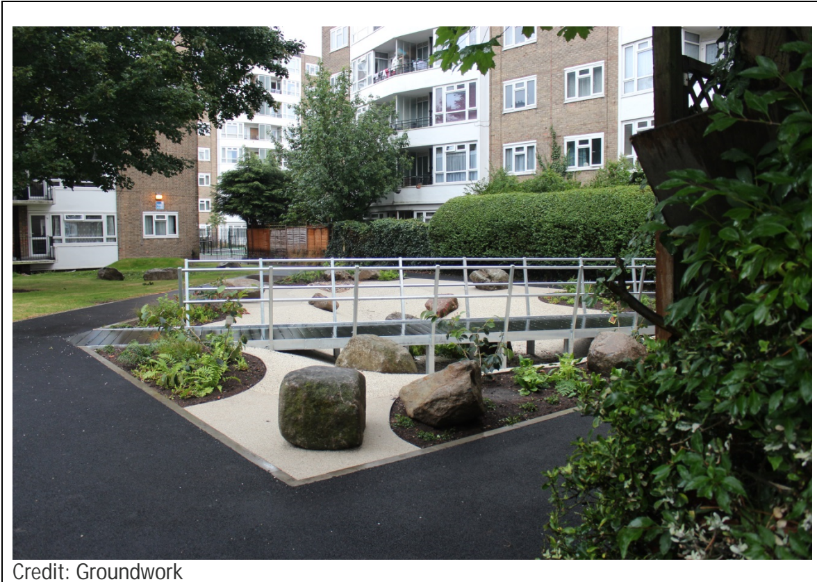
Figure 6: Groundwork estate retrofit project in Hammersmith & Fulham
