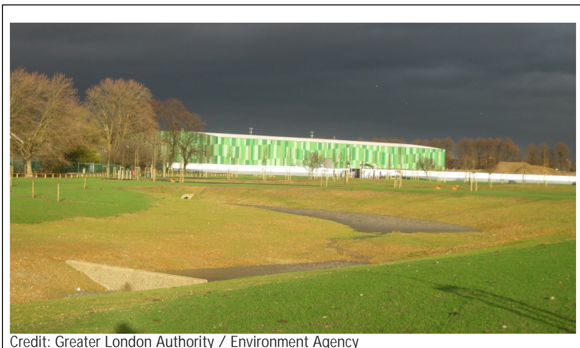
Figure 10: Swales installed at Mayesbrook Park, Barking and Dagenham
