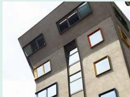
Roofline with greater extents than floors below
