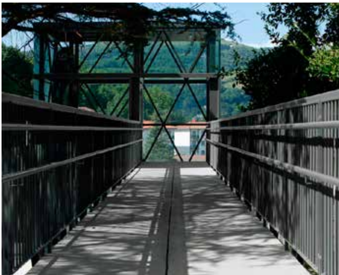
Bridge and lift, Galtzaraborda, Spain. VAUMM Architects
