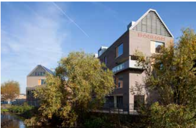
Roofscape Precedent: Thornsett Road, London
