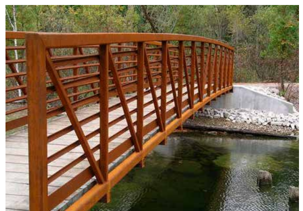
Bridge in weathering steel, Saskatoon, USA
