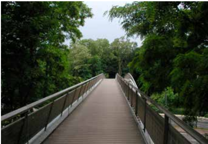
Bridge over Avenue Tervuren, Brussels. Pierre Blondel Architectes, Laurent Ney and Partners engineers
