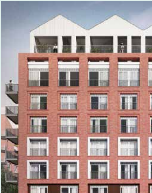
Regular pitched roofline set back from elevation
