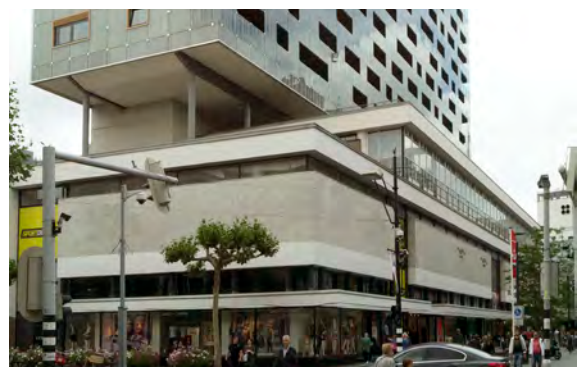
De Karel Doorman, Rotterdam Residential built on top of an existing shopping centre
