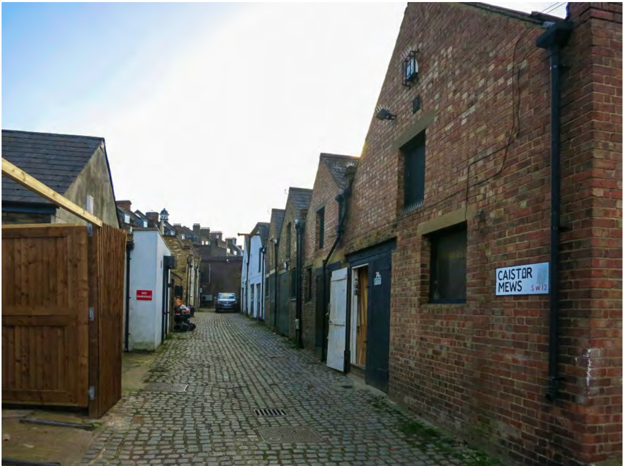
Light industrial units - Balham, Wandsworth
