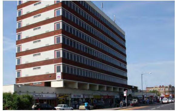
Colman Parade, Enfield Office space above retail
