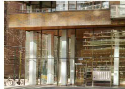
Large corner lobby
