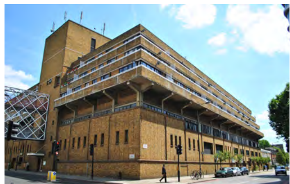
Warwick Road, Kensington & Chelsea Waste depot with residential above
