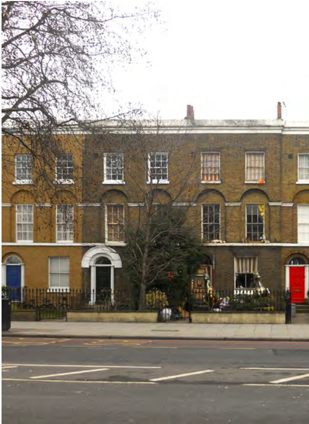
Mile End Road, Tower Hamlets
