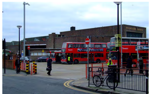
Hounslow Bus Garage, Hounslow Existing bus garage
