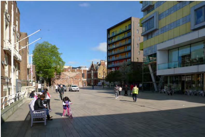
Barking Town Square, Barking & Dagenham
