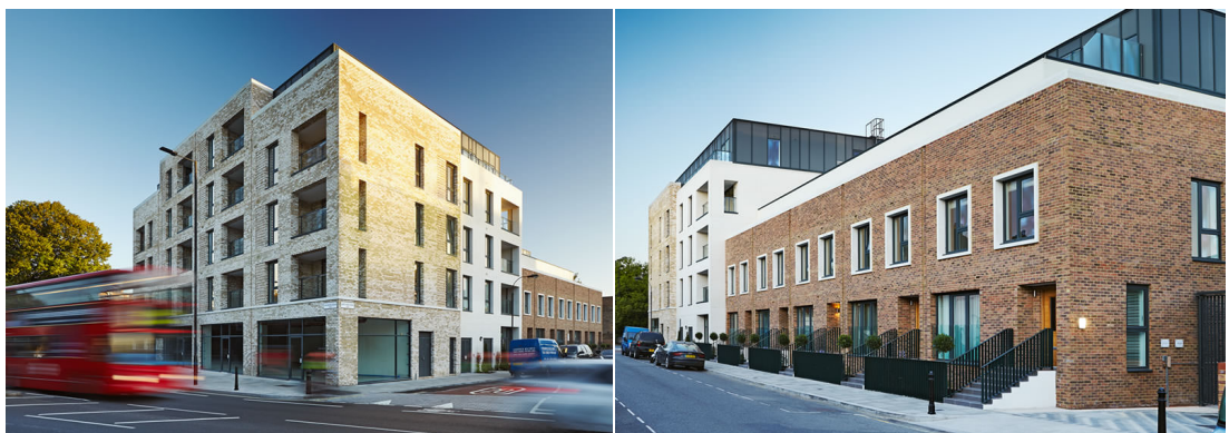
Figure 5.01 – Photographs of Parkside Place (© Linden Homes)
