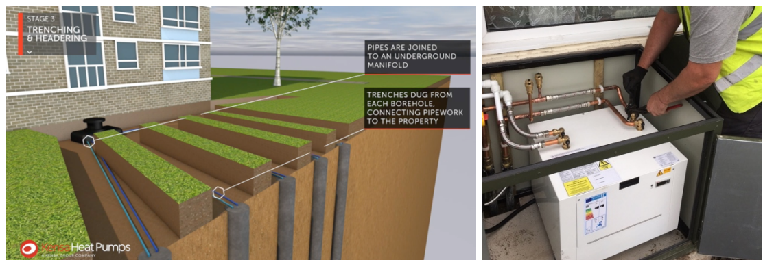
Figure 5.06 – Underground water loops (left) and individual ‘Shoebox’ heat pump (© Kensa)
