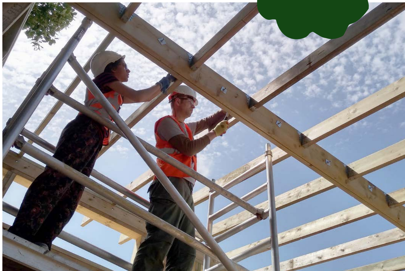
Photo: RUSS Ladywell Self-Build Community Space. Image courtesy of Graziano Milano.
