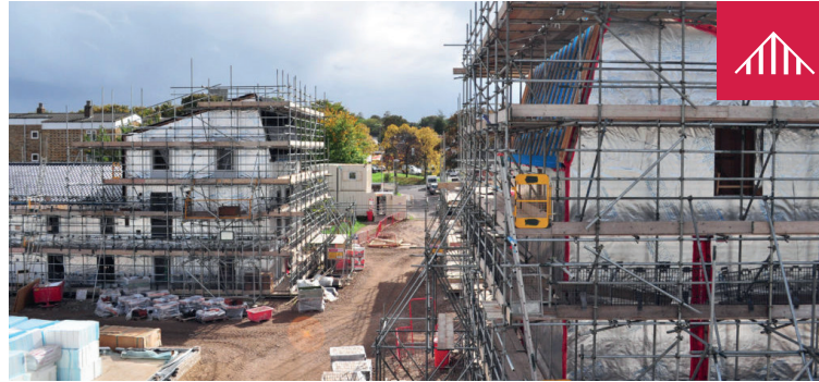
Category 2b. MMC – Cygnum for Norwich City Council, Goldsmith Street
