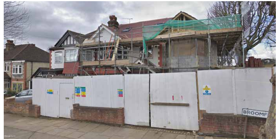
Ongoing flat conversion at 58 Broomfield Avenue.
