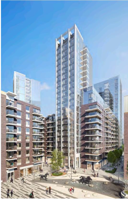
GOODMANS FIELDS, by Lifschutz Davidson Sandilands for Berkeley Homes, Tower Hamlets. Status: completed.
