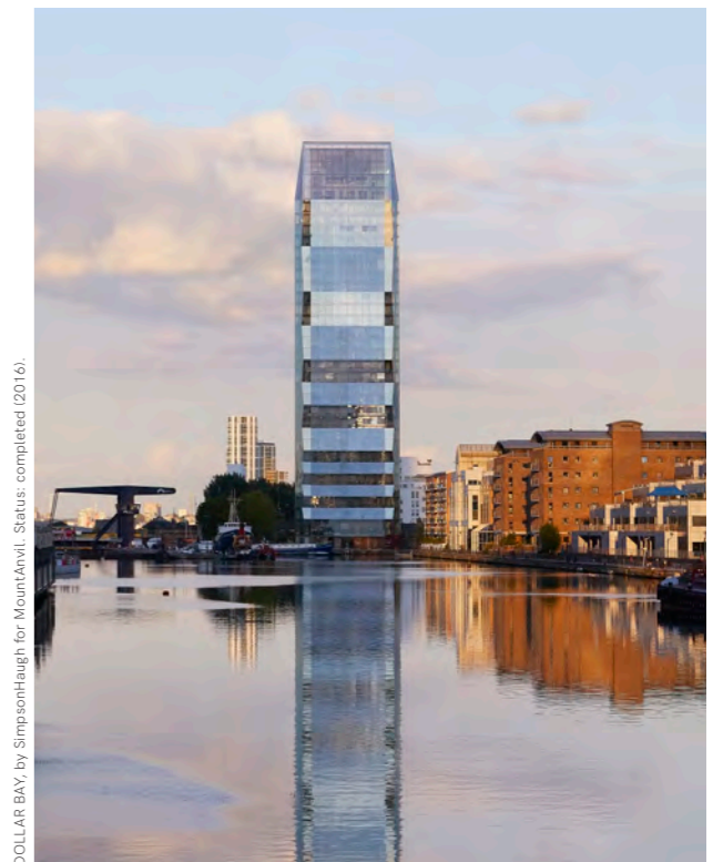
ONE BLACKFRIARS, by SimpsonHaugh for BerkeleyGroup. Status: under construction.
