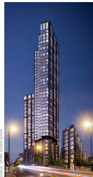
250 CITY ROAD, by Foster + Partners for Berkeley Homes, Islington. Status: under construction.
