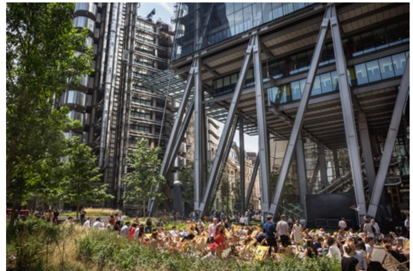
The Leadenhall Building, City of London
