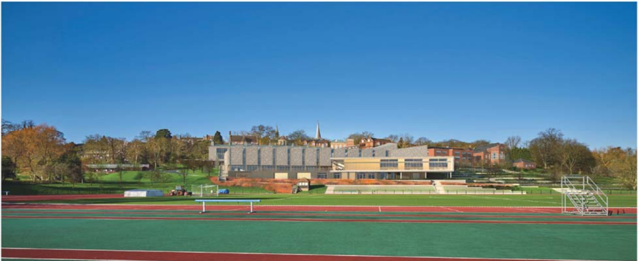
View from far side of the Athletics Track looking north east
