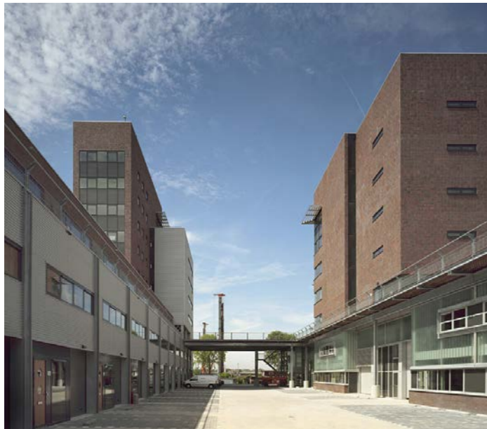
Stacked industrial - Steel frame KaaP Noord, Amsterdam, VSAP Architects
