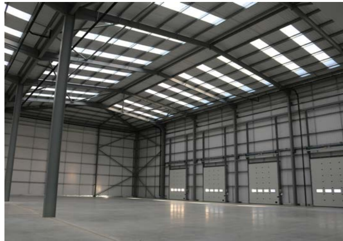
Single storey - Steel frame Unit 2, Origin, Park Royal, Segro
