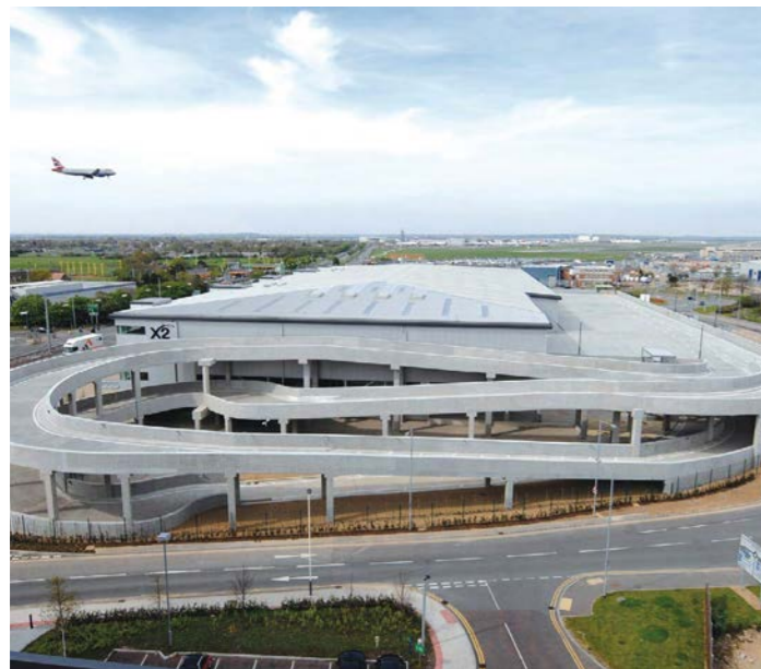
Stacked industrial - Steel frame with concrete ramp X2 Warehouse Hatton Cross, Cornish Architects
