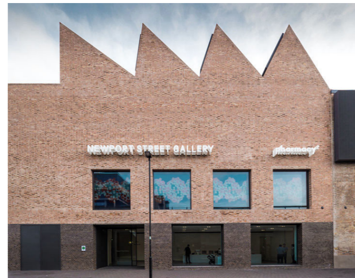
Newport Street Gallery, Caruso St John
