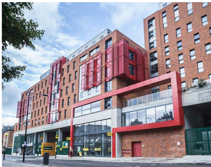
Mixed industry - residential - Concrete frame Travis Perkins Kings Cross, Cooley Architects
