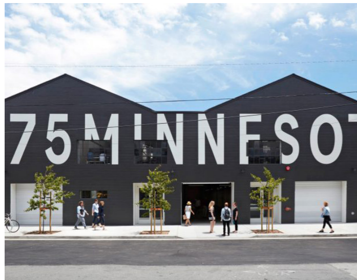
Minnesota Street Warehouse, Jensen Architects
